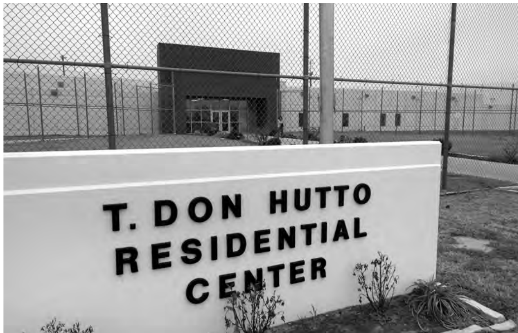
This former jail in Taylor, Texas, now houses about 400 immigrant detainees from more than two dozen countries.
